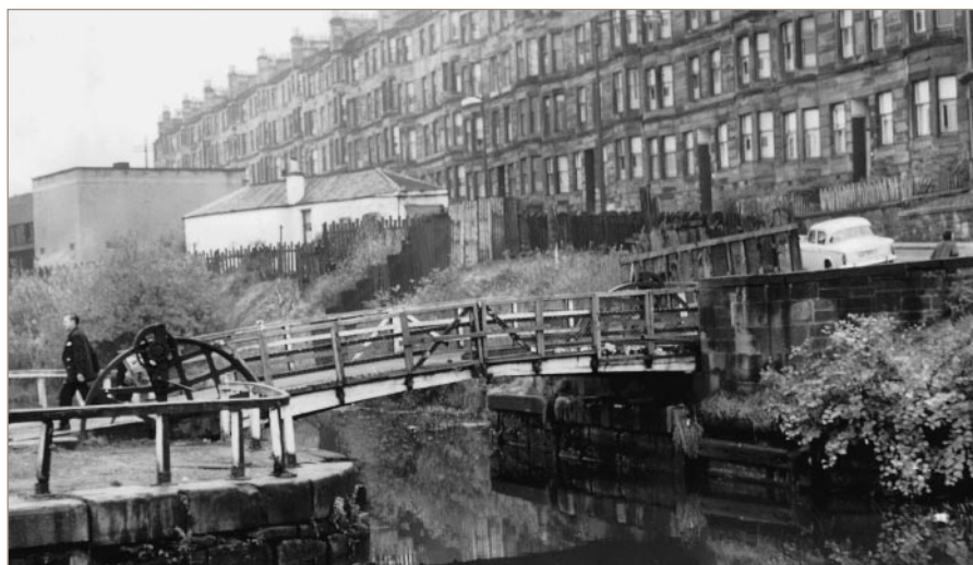
Fig. 9. Early 19th century replacement cast-iron and timber bascule bridge at Firrhill in Glasgow, c.1960 35
